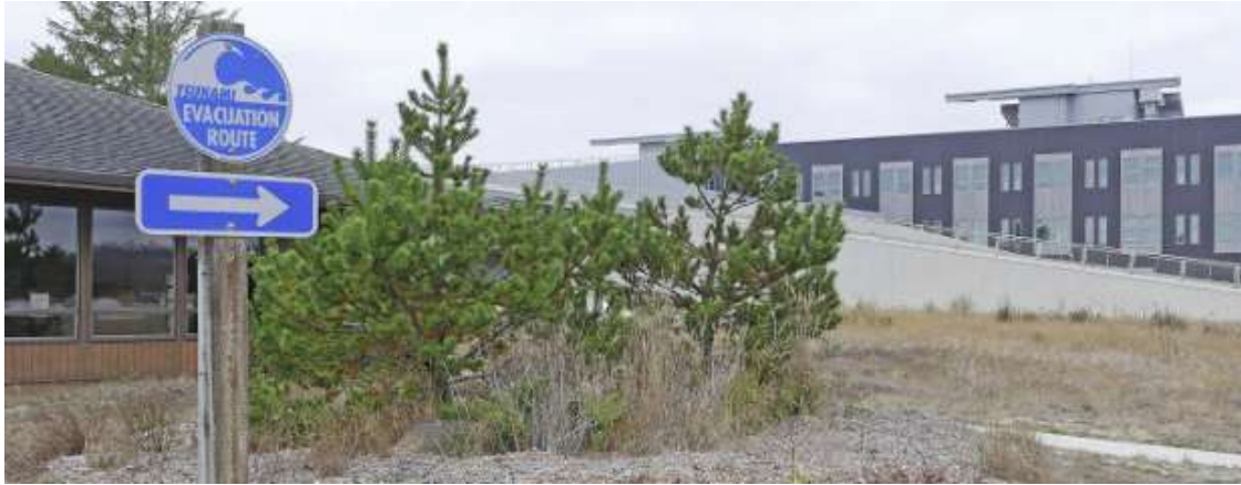
Oregon State University's Hatfield Marine Science Center in Newport, OR (pictured) has an integrated tsunami vertical evacuation structure built into the building. Photo Credit: Oregon State University.
