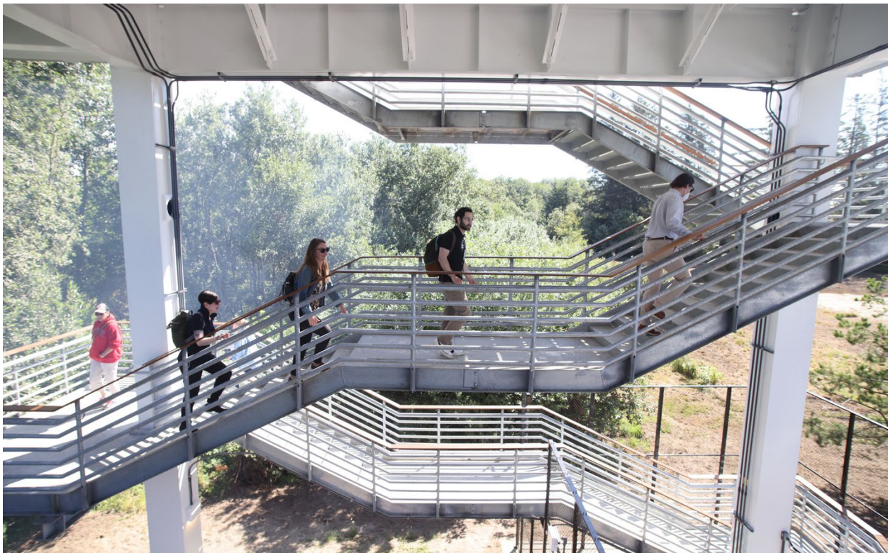
Figure 3. Staircase leading to the refuge platforms on the tsunami vertical evacuation tower built in Tokeland, Washington, by the Shoalwater Bay Indian Tribe. (Photo: Washington State Emergency Management Division)
