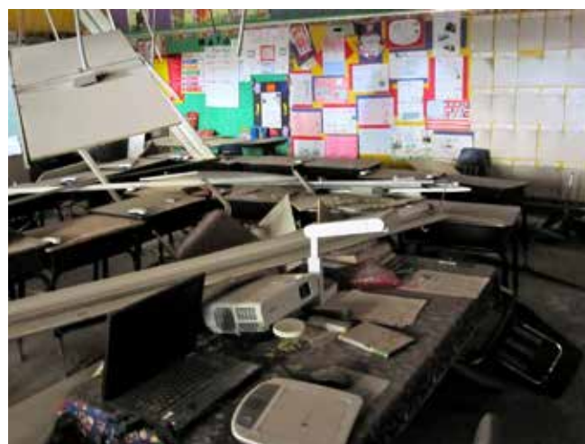
Figure 88. The 2010 Baja California M7.2 earthquake caused extensive damage to Jefferson Elementary School in Calexico, California, such that the school was closed for the remainder of the semester. Interior damage and fallen items could injure or kill students and faculty. Photo: Kelly B. Hutson.
