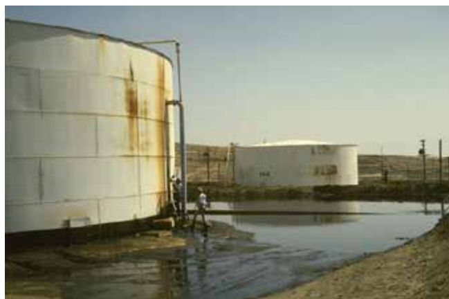
Figure 100. Shaking from the 1983 M6.5 Coalinga earthquake caused the pipe connections to break at a Chevron facility. Oil spilled out of the damaged connection, but was retained by dikes. Photo: Karl V. Steinbrugge.
