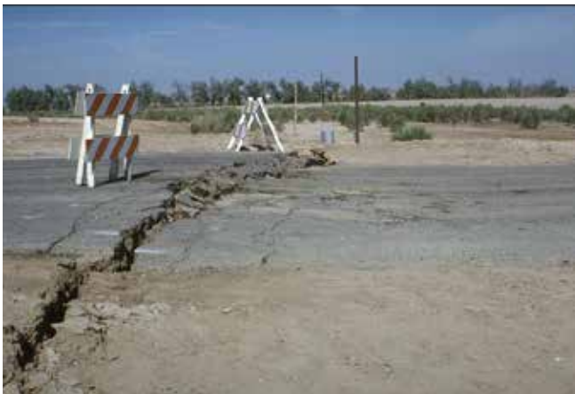
Figure 19. A M7.0 earthquake in California caused medium damage to roadways, with three to twelve inches of vertical displacement dissecting the road. This type of damage can be patched with an asphalt concrete overlay. Photo: Karl V. Steinbrugge, HITRAC.
