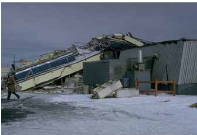
Figure 36. The Great Alaskan Earthquake in 1964 caused this reinforced concrete-framed control tower to collapse at the Anchorage International Airport. Photo: Karl V. Steinbrugge.
