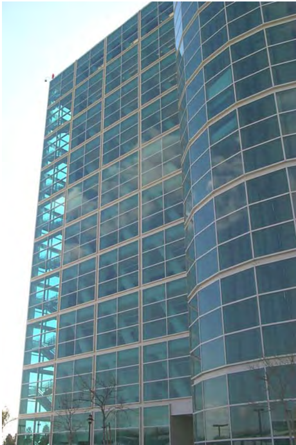
Figure 5-5 Exterior view of 3703 Roxbury Street.
