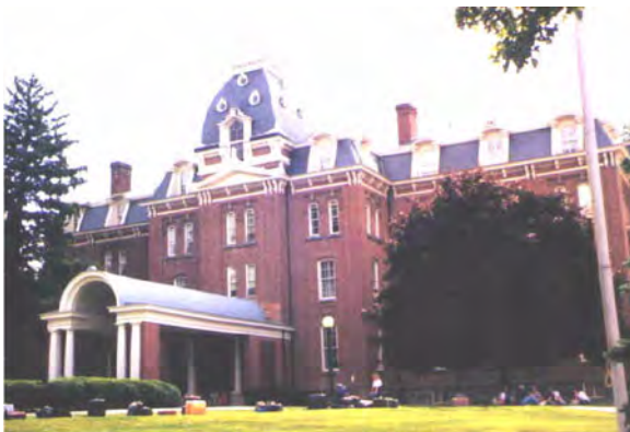
Figure E-50 East coast URM bearing-wall building.
