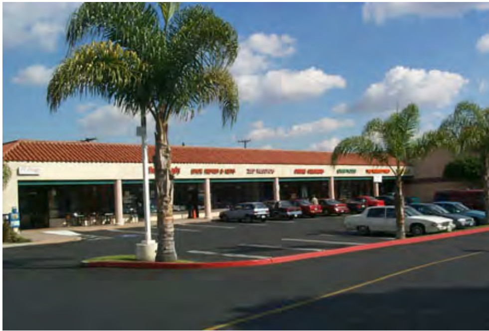
Figure 5-14 Exterior view of 1450 Addison Avenue.
