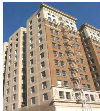
Figure E-33 Concrete frame with URM infill.
