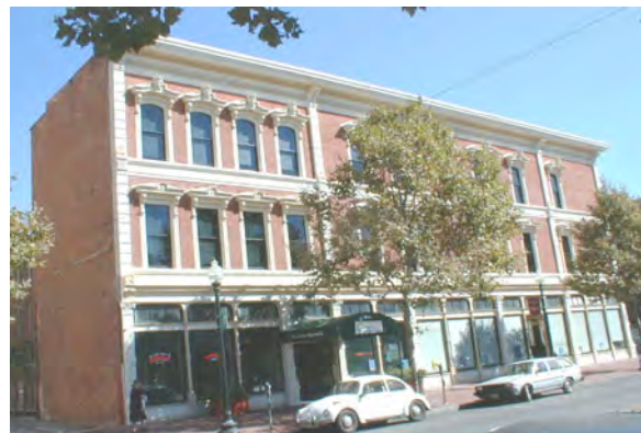
Figure E-51 West coast URM bearing-wall building.
