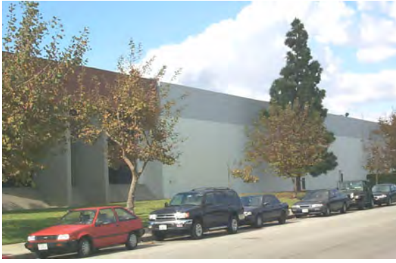
Figure E-36 Tilt-up industrial building, 1970s.
