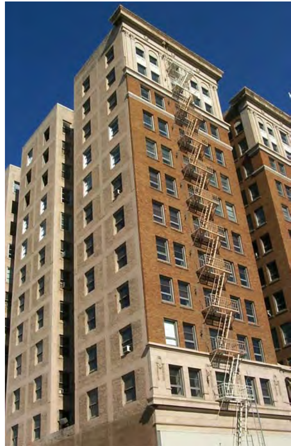
Figure 5-9 Exterior view of 3711 Roxbury.
