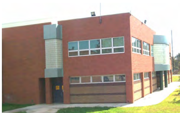
Figure E-46 Modern reinforced brick masonry.
