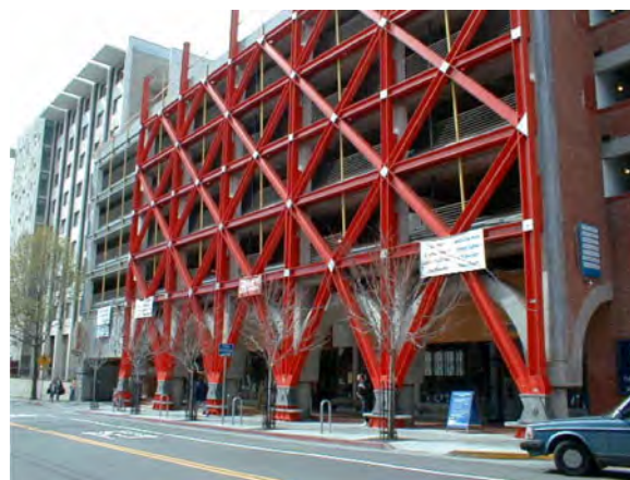
Figure E-15 Rehabilitation of a concrete parking structure using exterior X-braced steel frames.
