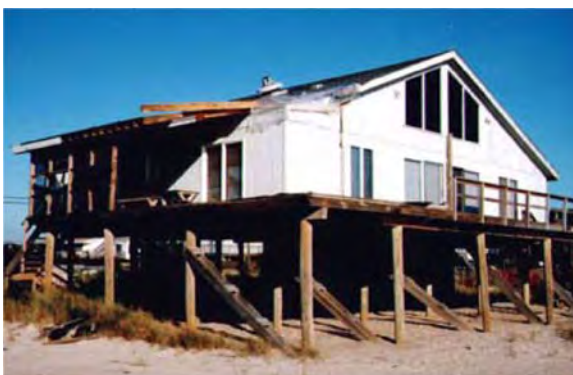
Figure E-6 Timber pole framed house.
