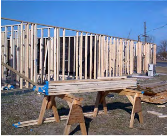
Figure E-4 Stud wall, wood-framed house.
