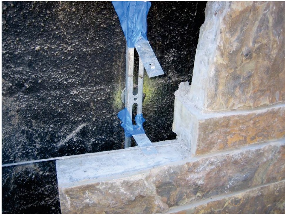
Figure 3-6. Brick veneer cladding being installed and securely attached to withstand earthquake shaking. Cladding should be designed and constructed to withstand earthquake shaking in Oregon (Source: FEMA, 2012).
