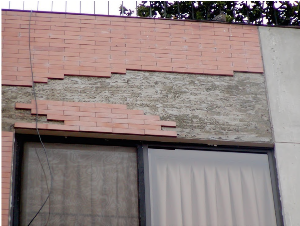
Figure 3-5. This building's brick veneer was not securely attached and was shaken loose in an earthquake (Source: FEMA, 2012).
