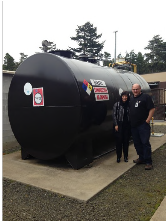
Figure 3-13. On-site emergency fuel tank.
