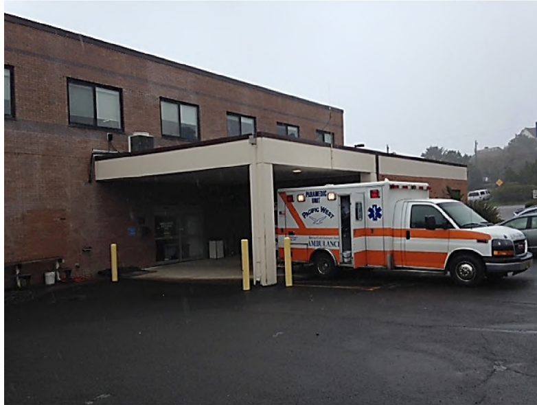
Figure 3-7. Heavy building cladding near hospital egresses should be able to tolerate earthquake shaking. Cladding installed before the mid-1990s should be evaluated for seismic hazards and, if needed, mitigated.
