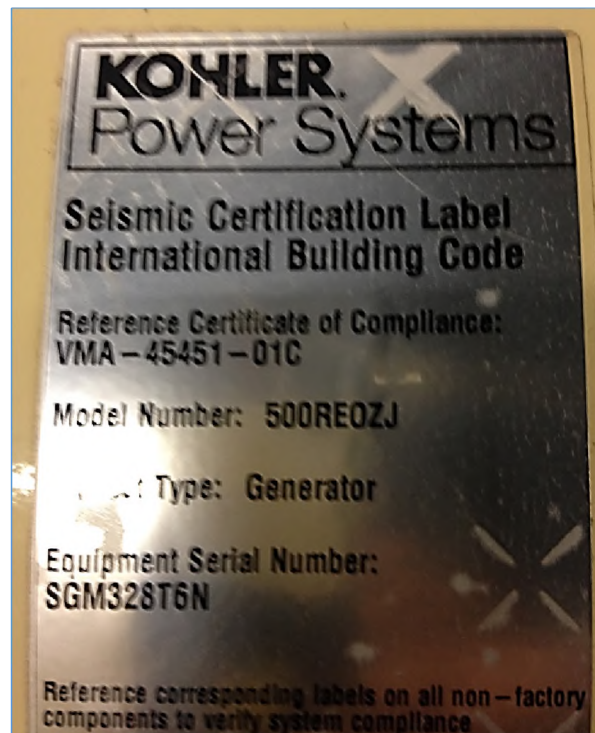
Figure 3-12. Seismic certification label attached to emergency generator shown in Figure 3-11.
