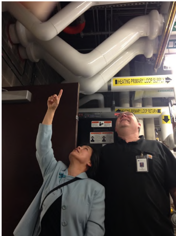
Figure 3-4. Flexible connections of utility pipes that allow for movement from earthquake shaking have been designed and constructed at the connection between two buildings (Photo credit: Deanna Henry, ODOE).
