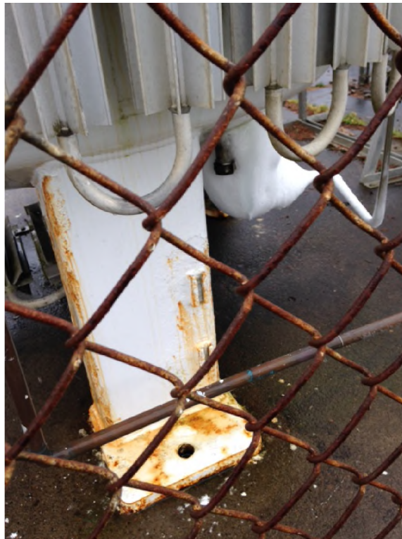
Figure 3-10. Close-up of medical gas tank in Figure 3-9 showing inadequate anchorage.
