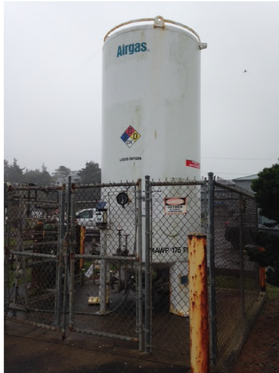
Figure 3-10. Close-up of medical gas tank in Figure 3-9 showing inadequate anchorage.
