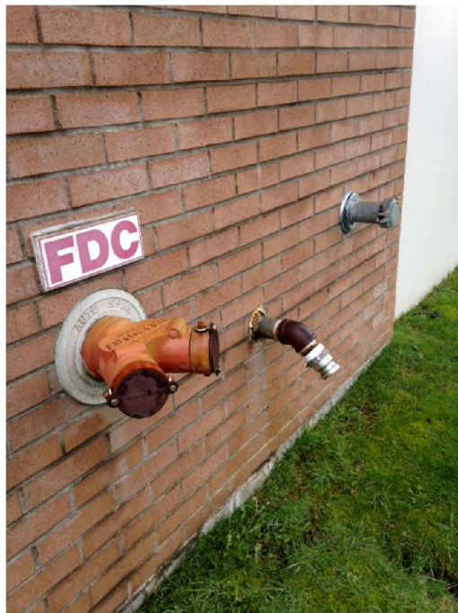
Figure 3-8. Safety related utilities can be damaged by seismically vulnerable building cladding. Cladding installed before the mid-1990s should be evaluated and, if needed, mitigated.
