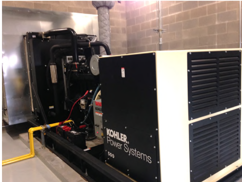
Figure 3-11. Emergency generator, which is part of the emergency power system. This generator has been seismically certified, as shown in Figure 3-12.
