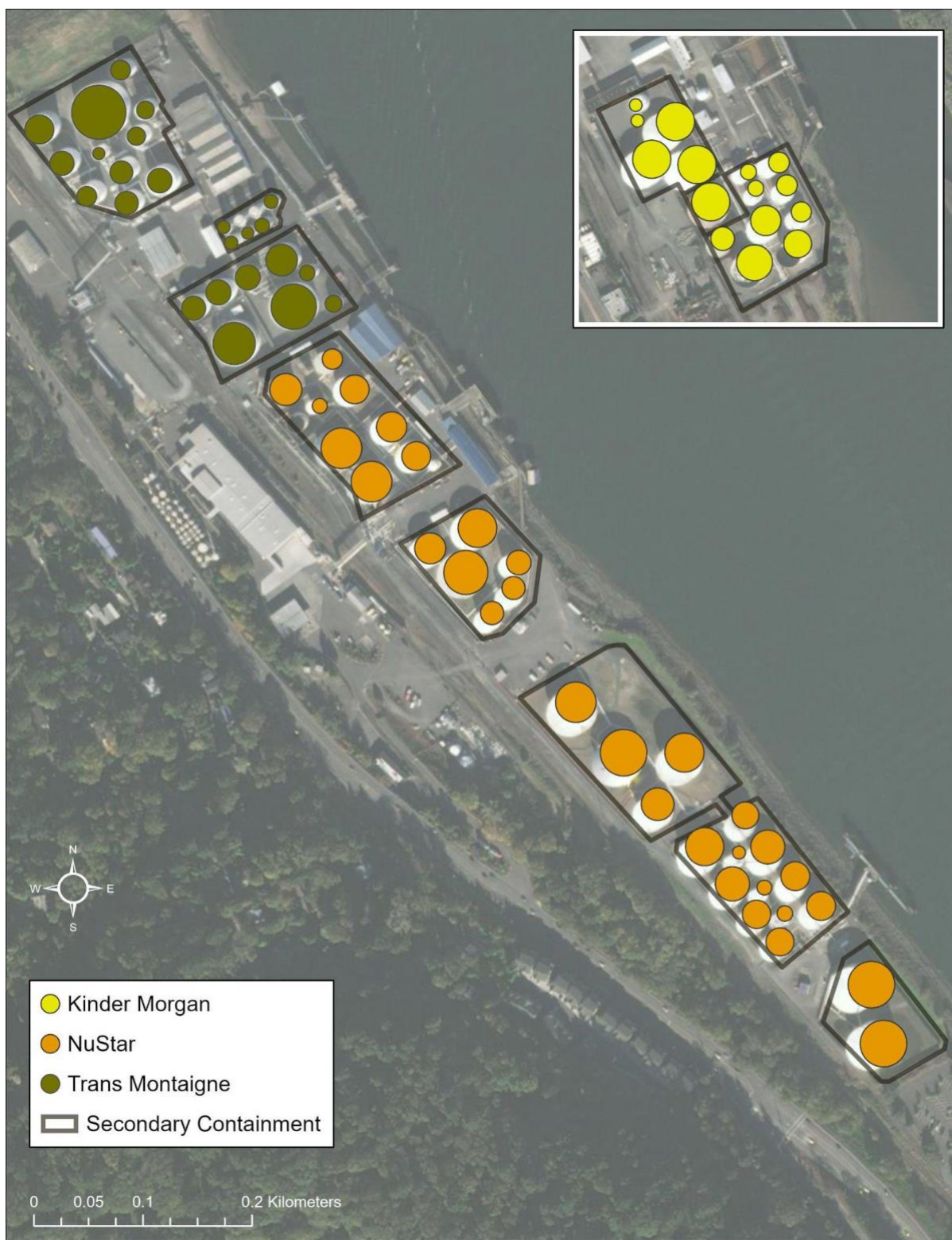
Figure 8-2. Overview of the upper CEI Hub located at Linnton terminal.
