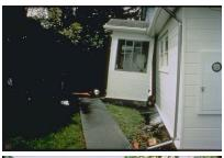
**Petrolia residence shifted on foundation** This Petrolia residence shifted on its foundation causing the porch to separate from the house. Wooden skirting along the bottom of the house shows the direction of movement of the house on the foundation. Photograph credit: Lindie Brewer, U.S. Geological Survey.
