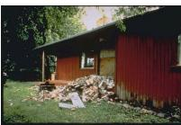
Chimney damage in Petrolia This brick chimney, typical of many others in Petrolia, was toppled due to the severe earth shaking. Other chimneys (even those with steel rods) were broken, or cracked. The inside fireplace in this house was also shattered. Photograph credit: Lindie Brewer, U.S. Geological Survey.
