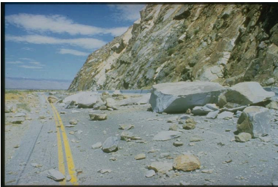
Rockfall on Highway after 1986 Palm Springs Earthquake Earthquake of July 8, 1986, Palm Springs, California. This rockfall on the highway is just one of many landslides that occurred in the Palm Springs, California, area. Such rockfalls can temporarily block roads and highways and hinder the movement of emergency vehicles. [Photo credit: Bay Area Regional Earthquake Preparedness Project.]
