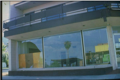
Damage to Display Window, 1986 Palm Springs Earthquake Earthquake of July 8, 1986, Palm Springs, California. A broken display window in downtown Palm Springs. Display windows often break in moderate magnitude earthquakes since the window occupies a large, structurally-unsupported area of the building subject to torsional forces. [Photo credit: Bay Area Regional Earthquake Preparedness Project.]
