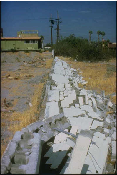
Collapsed Concrete Block Fence Due to 1986 Palm Springs, CA Earthquake Earthquake of July 8, 1986, Palm Springs, California. This concrete block fence near a trailer park collapsed during the quake. Such fence failures were common. Note bent reinforcing rod. [Photo credit: Bay Area Regional Earthquake Preparedness Project.]
