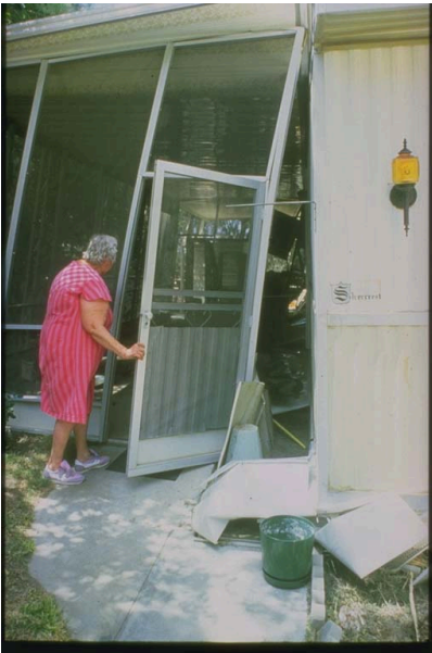
Porch Damage, 1986 Palm Springs, CA Earthquake Earthquake of July 8, 1986, Palm Springs, California. This porch was separated from the trailer and damaged by the quake. Trailers incurred more structural damage than any other type of structure in this earthquake. [Photo credit: Bay Area Regional Earthquake Preparedness Project.]
