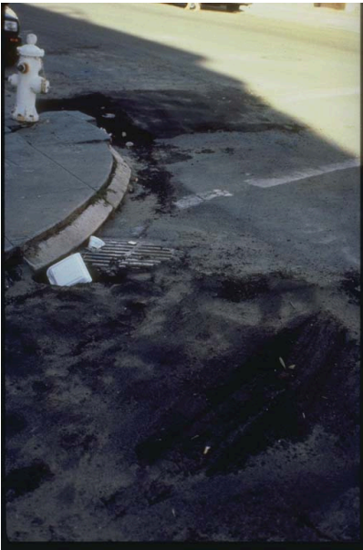
Evidence of Liquefaction in the Marina District, San Francisco The fine sand deposited near the curb is evidence of the liquefaction that took place in the Marina District. Some sand boils in the area spewed forth charred wood and other debris, remnants of the San Francisco that was destroyed by earthquake and fire in 1906. [Photo credit: D. Perkins, U.S. Geological Survey.]
