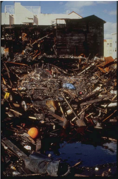
Rubble Left after Fire in Marina District Rubble after the fire at North Point Street and Divisadero in the Marina District. As in 1906, water mains failed and fires in this area could not be fought with city water. Water was pumped from a fireboat to extinguish this fire. [Photo credit: D. Perkins, U.S. Geological Survey.]
