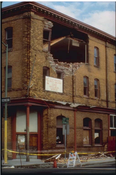
Damage to Top Floor of Clay Building, Oakland, California Damage to the upper floor of the three-story Clay Building at the corner of 10th and Clay Streets in Oakland, California. [Photo credit: C. Stover, U.S. Geological Survey.]
