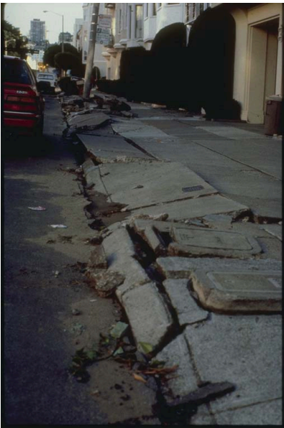
Sidewalk Damage Produced by Liquefaction, Marina District, San Francisco View south on Webster Street in the Marina District. Sidewalk damage is the result of liquefaction of the land fill upon which the area was built. Note the upheaved section in the background near the pole. The manmade fill beneath the Marina District was permanently deformed by liquefaction. Structures resting on the fill had to accommodate the deformation. [Photo credit: D. Perkins, U.S. Geological Survey.]
