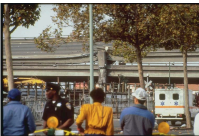
Side View of the Collapsed Section of Interstate 880, Oakland, California Side view of the collapsed Cypress section of the Interstate 880. Note the failed column support in the center of the photo and the ambulance to remove survivors. [Photo credit: C. Stover, U.S. Geological Survey.]
