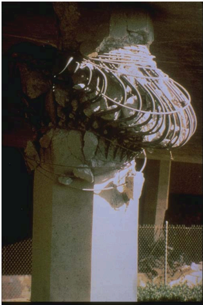
Failed bridge support, Northridge earthquake Bridge column supporting Interstate 10 (Santa Monica Freeway) at the La Cienega-Venice overcrossing failed in the 1994 Northridge earthquake. [Photo credit: M. Celebi, U.S. Geological Survey.]
