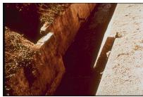
**Drain offset caused by seismic creep** Right-Lateral Strike-Slip Faults Drain offset produced by seismic creep along the San Andreas fault at the Almaden Winery in central California. The winery is also experiencing offset walls, bent and broken pipes, etc., due to seismic creep. Motion along the fault is mostly strike-slip. [Photo credit: University of California, Berkeley.]
